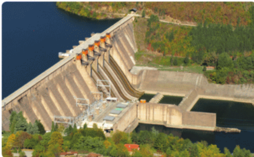
Water power plant
