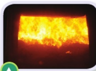
Figure 10.23 Waste being burned in an incinerator
