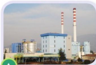
Figure 10.22 A waste incinerator
