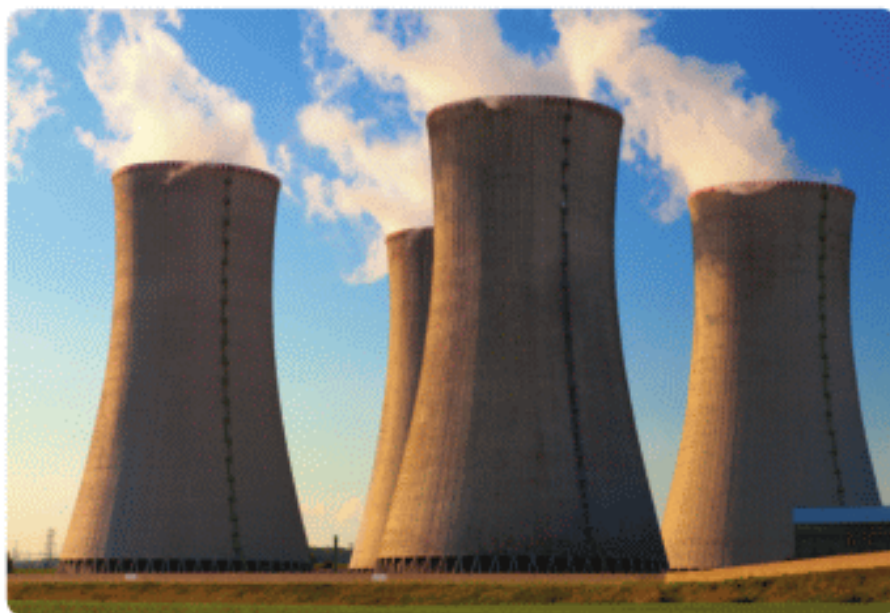
Nuclear power plant
