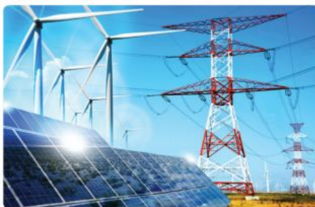
Modern electric grid lines
