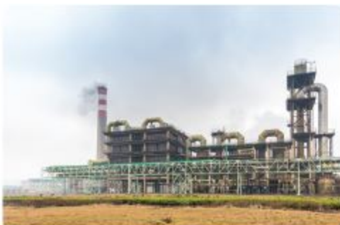
Sulfuric acid plant
