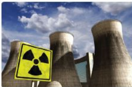
Nuclear power station
