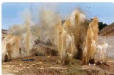
Shooting explosives in a stone quarry
