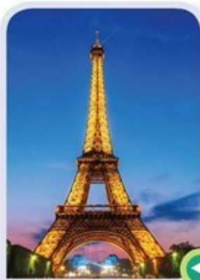
Figure 5.7 The Eiffel Tower is made of iron and needs repainting every seven years
