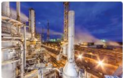
Nitric acid production on fertilizer plant
