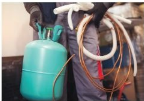
Removing gases from the freon tubes
