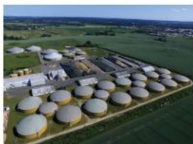
Big biogas plant
